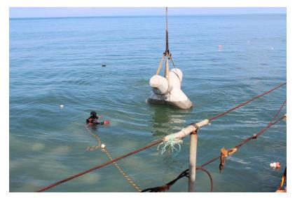
• The work was done using the following technique: tug 1500 strong, barge 3000 tonne PDM 13, crane 100 tonne, 2 self-propelled barges 1200 tons each, special diving boat (with baro camera), fully equipped team of divers and equipment for researching the bottom (echo sounder, scanner, video / camera)
